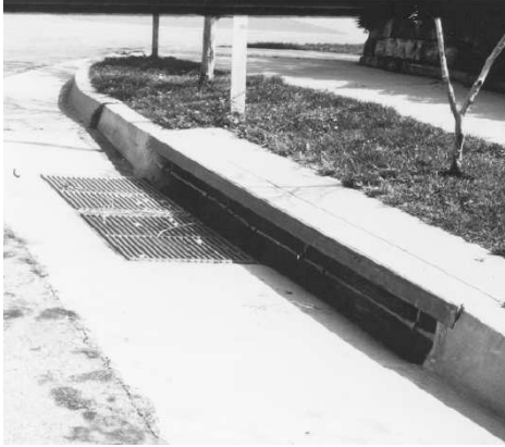
Figura 10.25 Boca de tormenta combinada (FHWA, Urban Drainage Design Manual)
