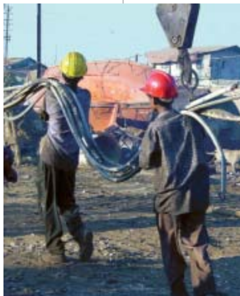
Workers at the Alang Sosiya ship-breaking yard, December 2001.
